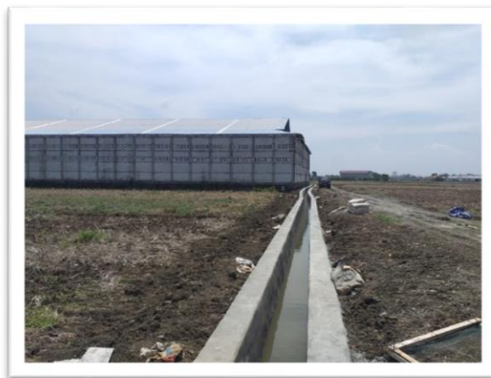
Gambar 3.4 Rehabilitasi drainase kauman (BANGUB)
