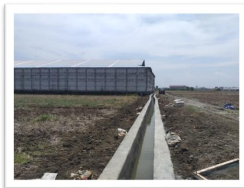
Gambar 3.4 Rehabilitasi drainase kauman (BANGUB)
