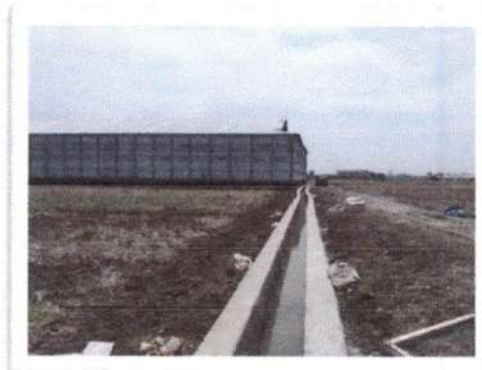
Gambar 3.4 Rehabilitasi drainase kauman (BANGUB)
